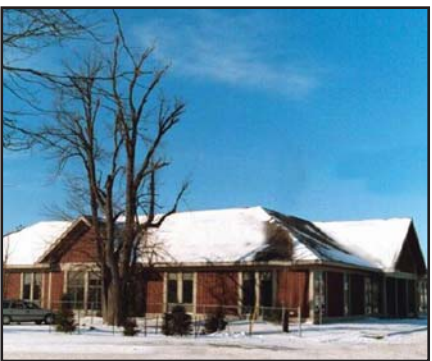
Merrickville District Community Health Centre, 10,000 square feet, $1.42 million, 1998-1999. A long-term land lease was negotiated with the Village of Merrickville-Wolford for a site adjacent to the community centre, municipal offices and fire station.
